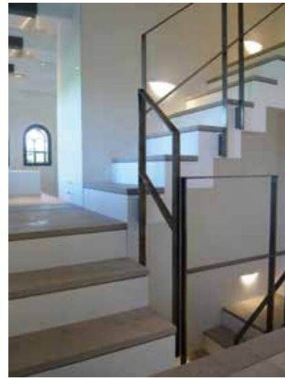
Solid structures: steel, oak – and tight project management on site
